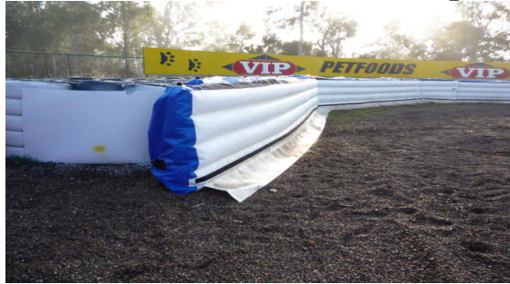
Airfence installed at T3, Queensland Raceway.
